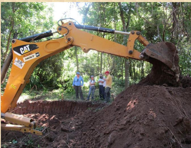
Backhoe at Cotton Field preparing a new area for excavation.
