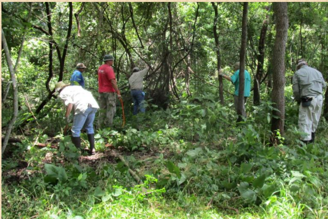
Cotton Field before – crew from HAS clears brush in preparation for bringing in a backhoe to scrape a larger area to excavate during field school.
