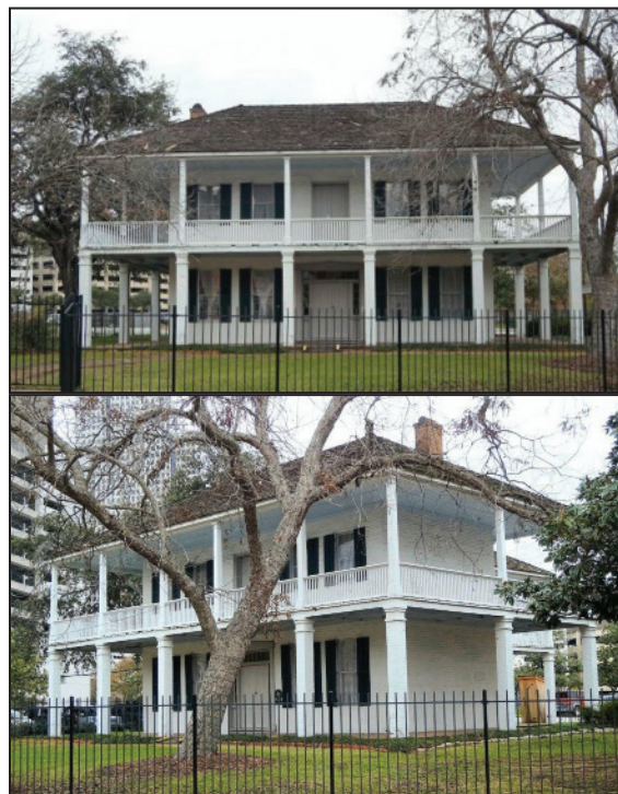
Figure 5a-b. Modern Kellum-Noble House Museum (5a - front view (top); 5b - side view (bottom)).
