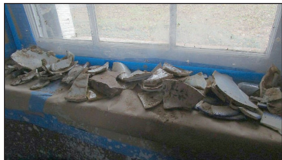
Figure 9. Broken ceramics found during restoration of the Kellum-Noble House by contractors and stacked on window sill.
