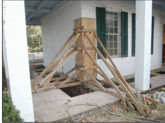
Figure 8. Shored up exterior wall.
