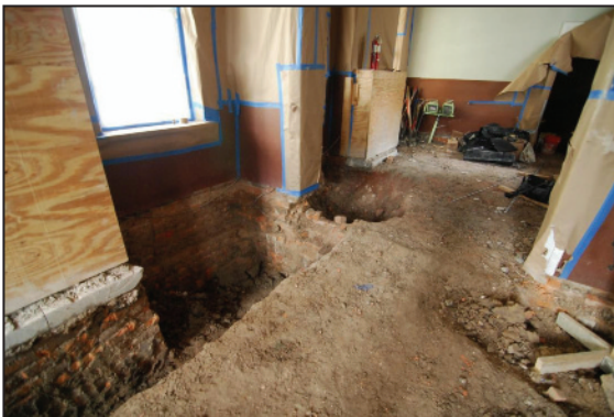
Figure 12. Flooring removed and foundations dug down (December 2014).
