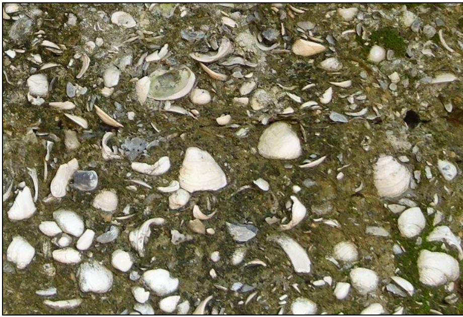
Figure 4: Rangia clam shells are the aggregate used in the concrete of the wall of the W. D. Cleveland and Company building. (Louis F. Aulbach).
