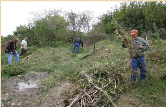
The crew stacking up brush to be hauled away.
